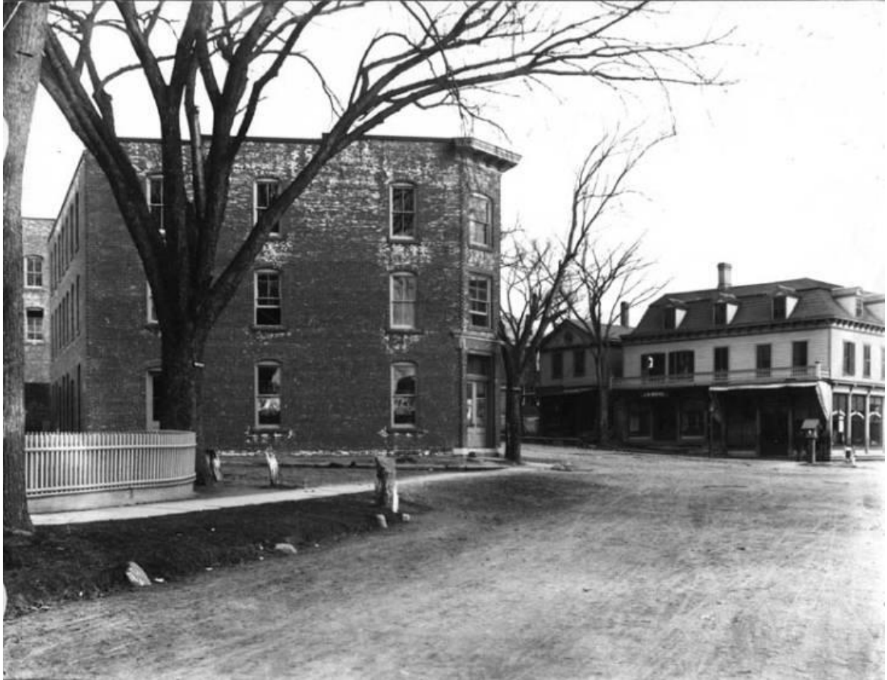
Hall Block and Jennings Building, Main and Harbor Rd Southport, CT 1896?
