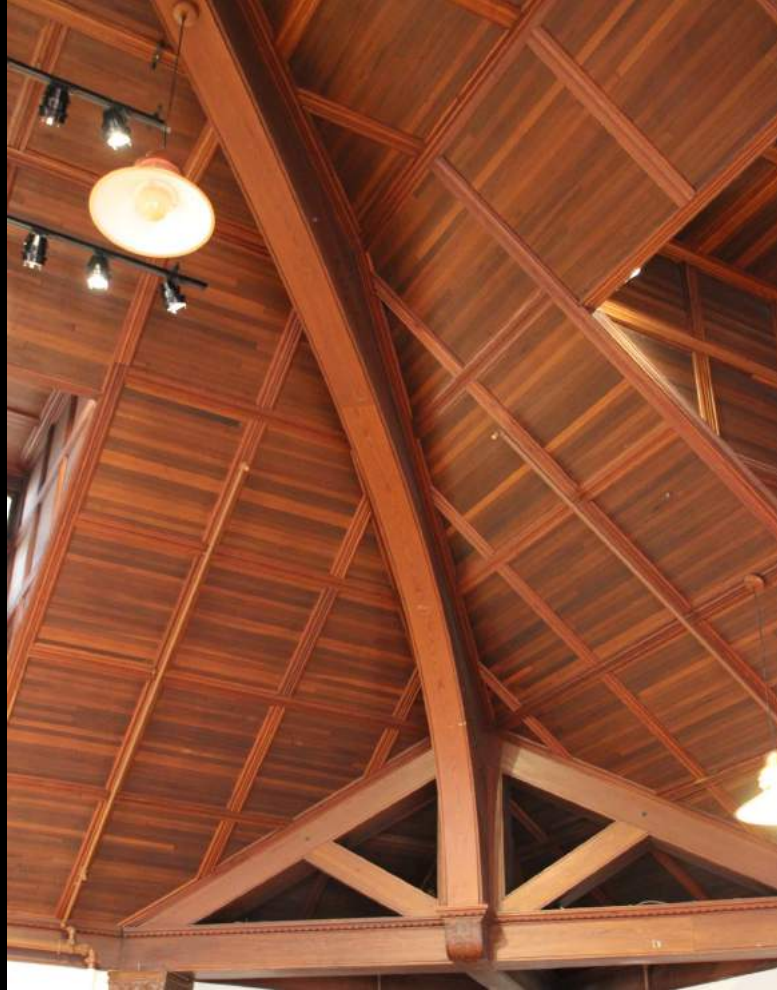
Auditorium Ceiling Detail
