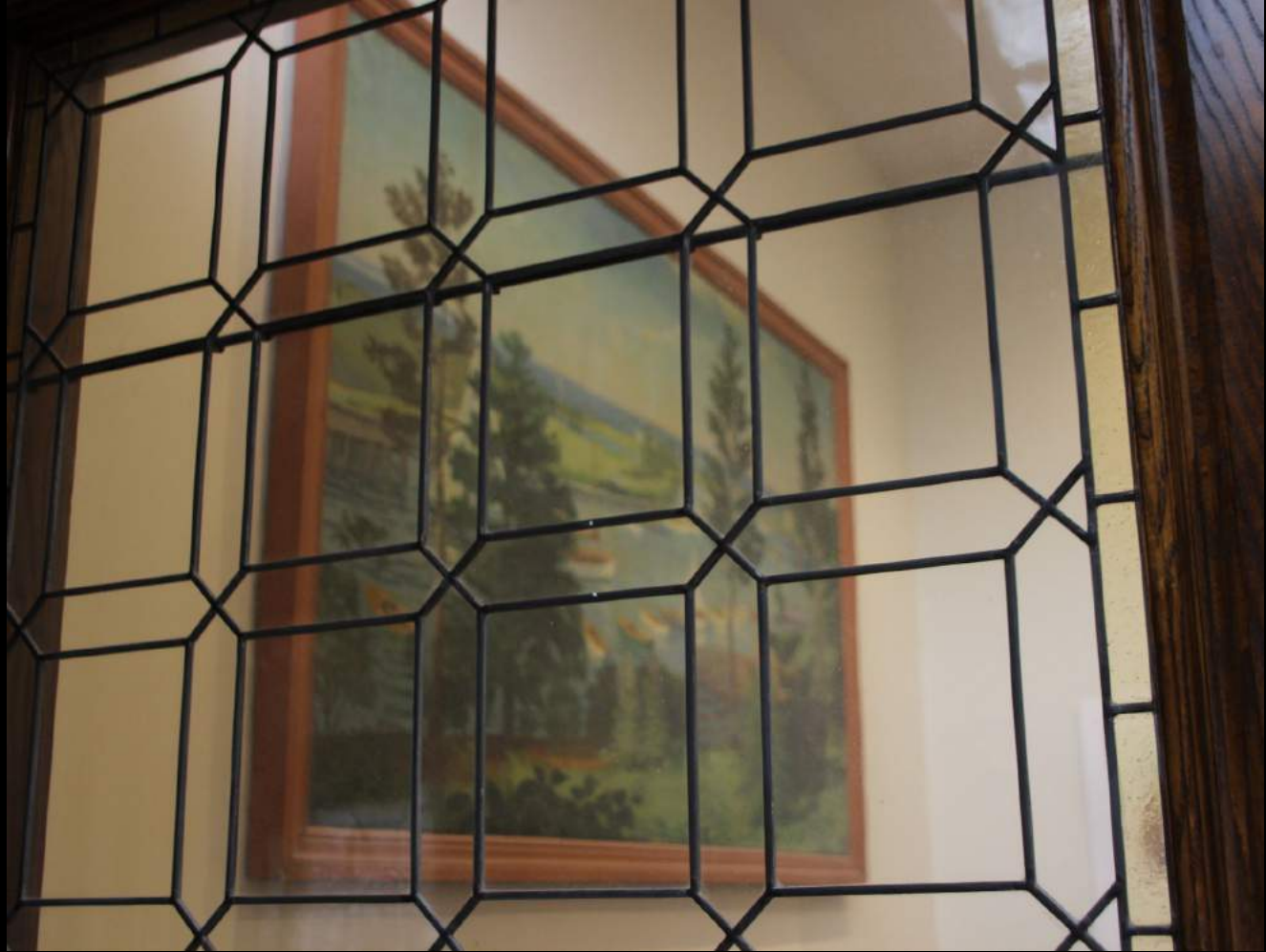
Foyer Window Detail
