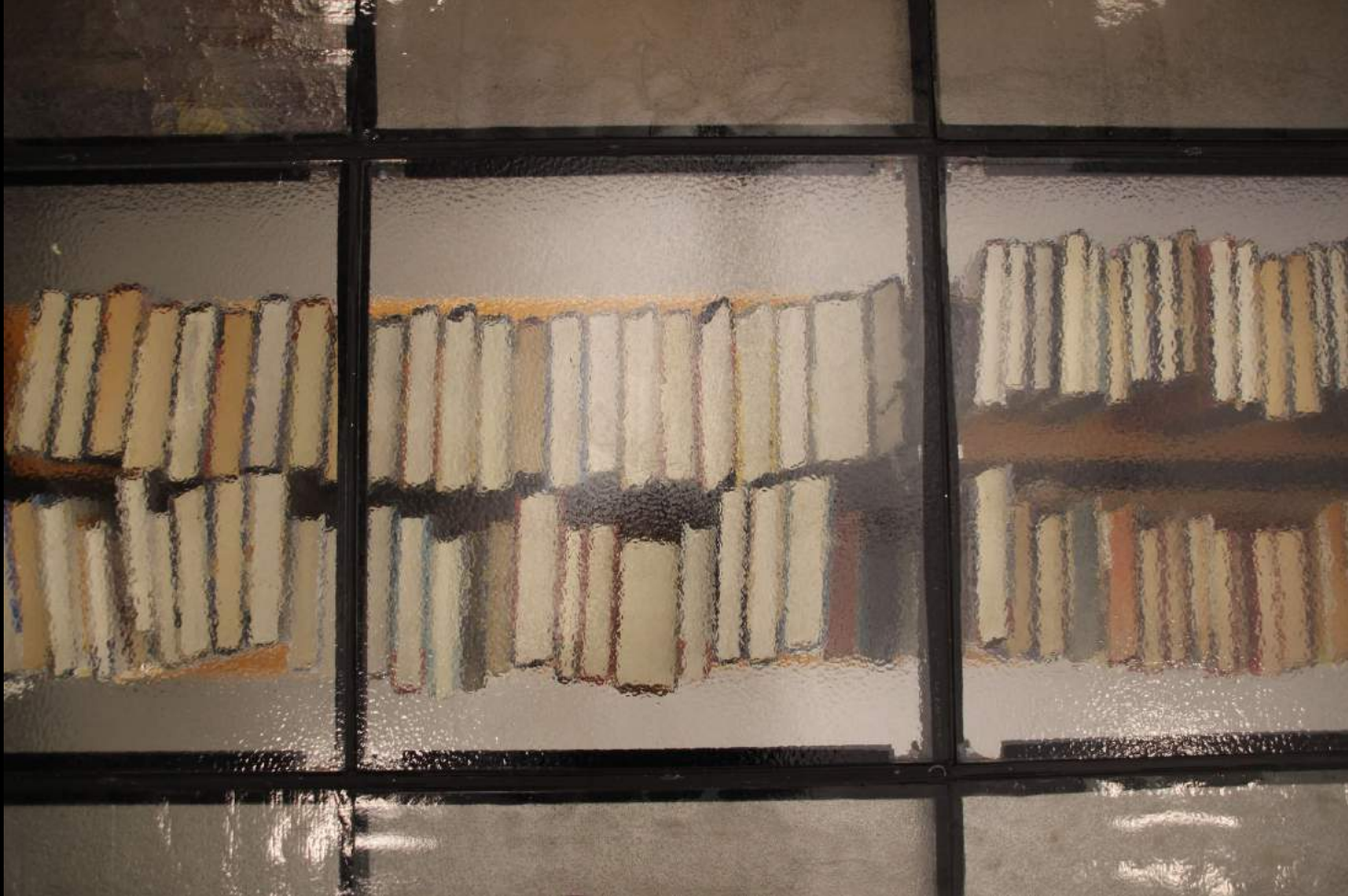
Mezzanine Detail Glass Floor
